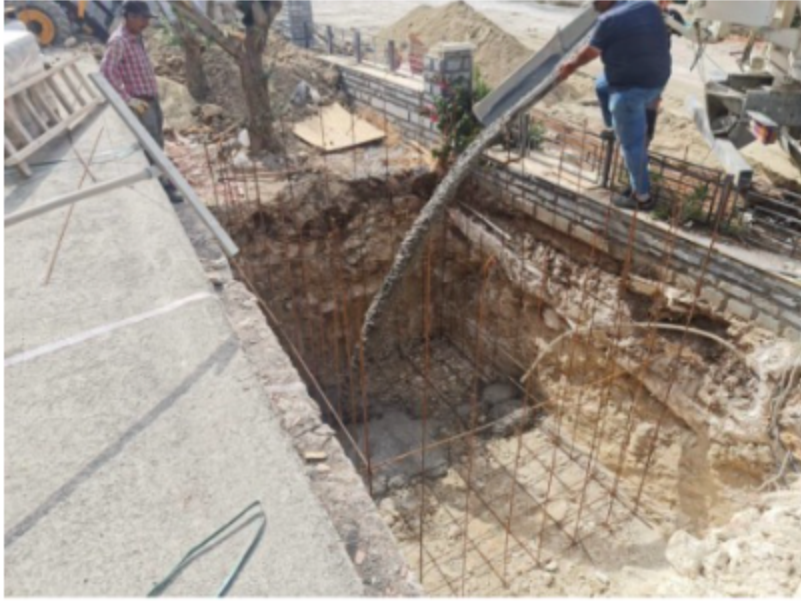
Figure 5. Residences that are not connected to existing wastewater infrastructure construct septic tanks beneath their houses; septic tanks are not regulated to ensure that proper sanitation practices are being followed. (Taken on July 2 at 6224 Sokak, No; 12, Yali Mahallesi, Izmir, Türkiye).
