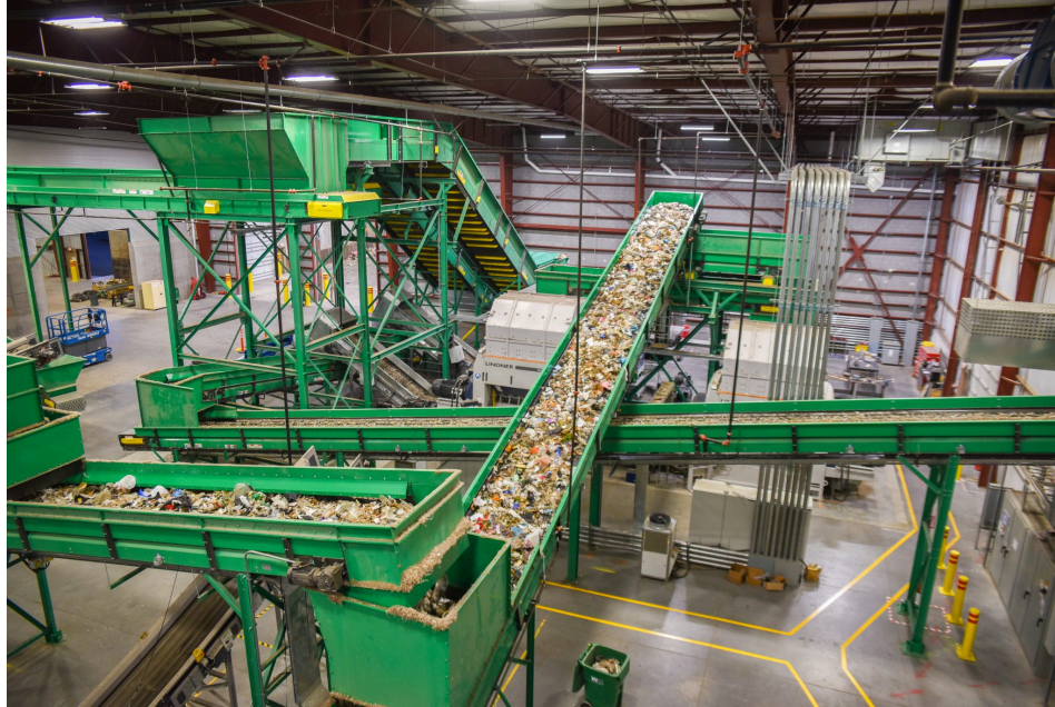
Figure 1.2.1: Material Recovery Facilities segregating general waste (Cambridge Companies, 2025)
