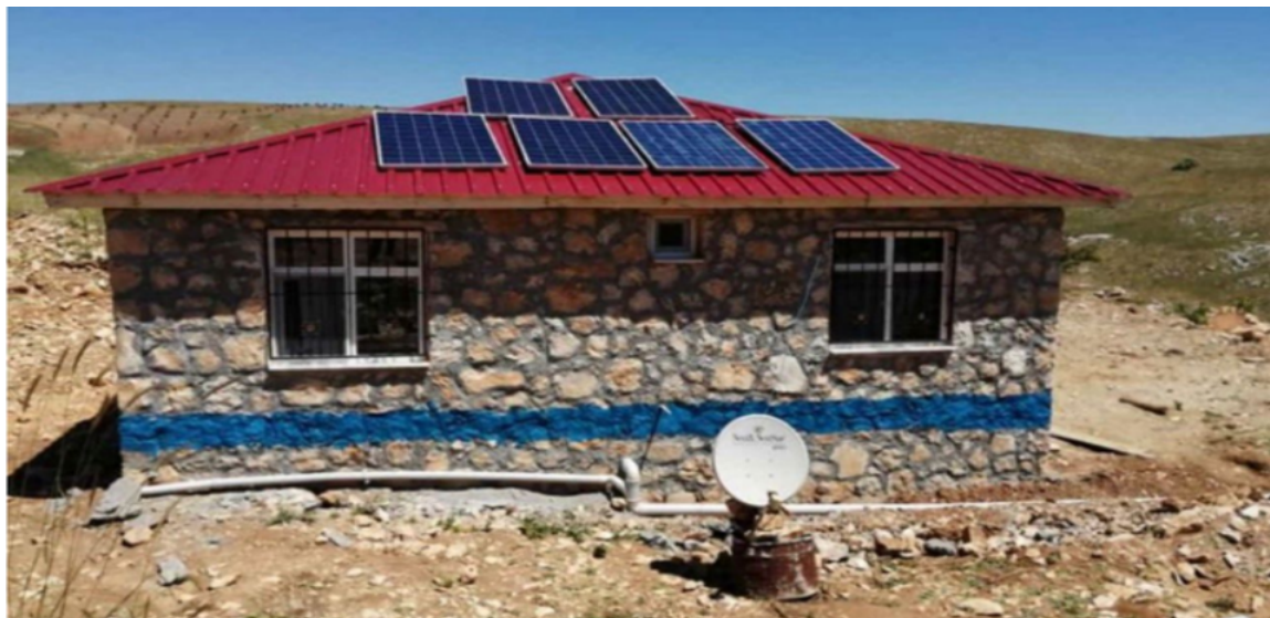
Figure 2. Off.grid infrastructure: The high thermal mass stone house constructed from cleared site rocks, equipped with a rooftop photovoltaic solar power system.
