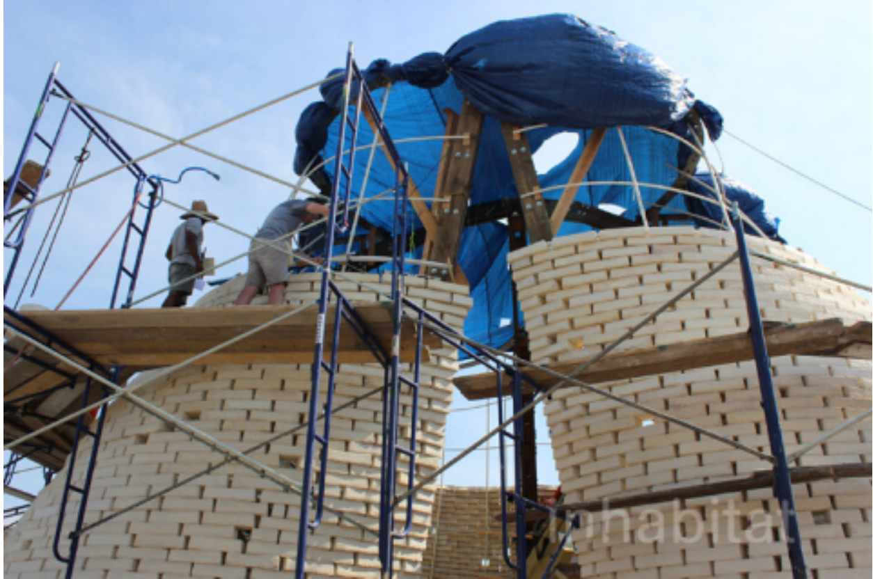
Figure 1. Hy-Fi Tower construction at MoMA PS1, New York, 2014.
