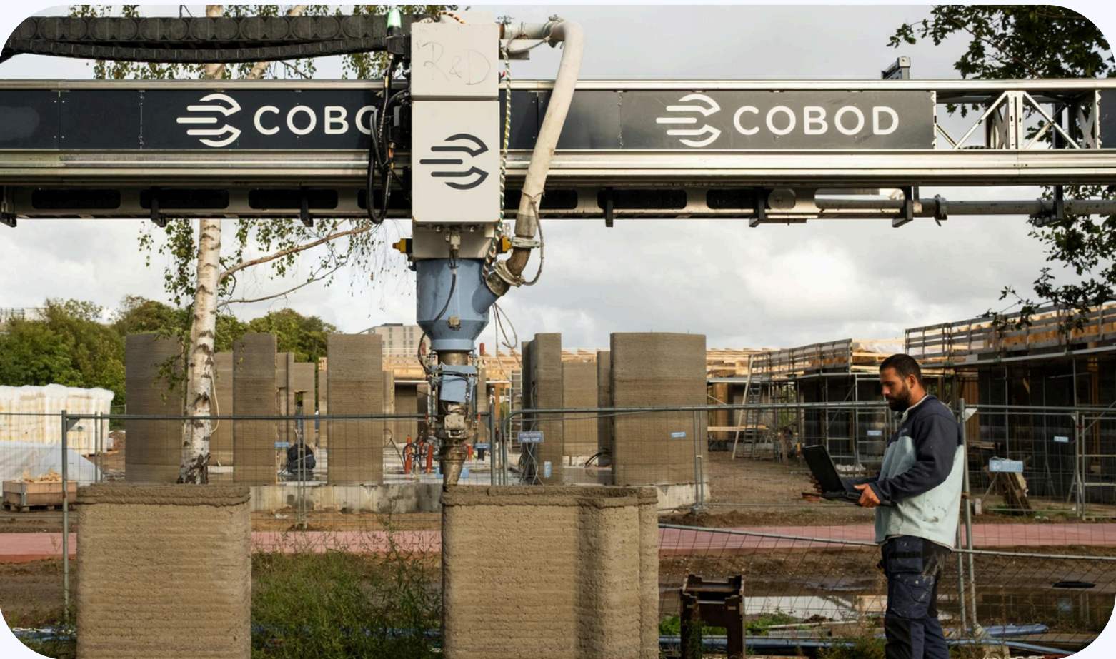
Robotic additive manufacturing in construction. Image: COBOD International [15]
